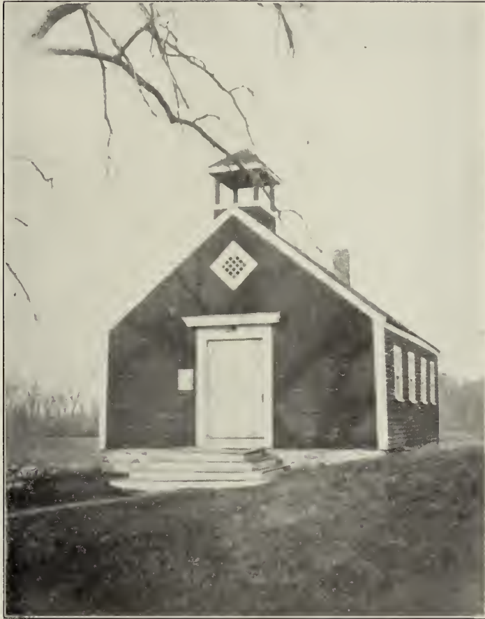
CHAPEL FIRST SCHOOL BUILDING AT DUMMER 1763
